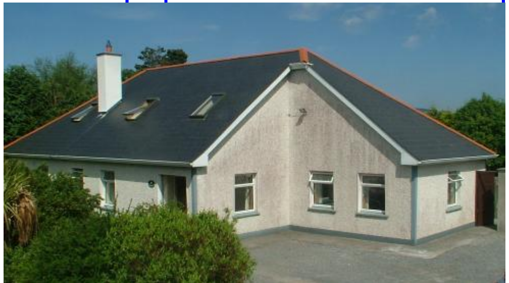
WOODHAVEN HOUSE BEFORE THE REFURBISHMENT
